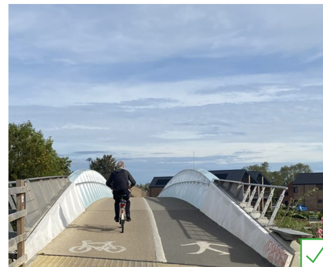
Bridge to provide access pedestrian and cycle access to Village 1
