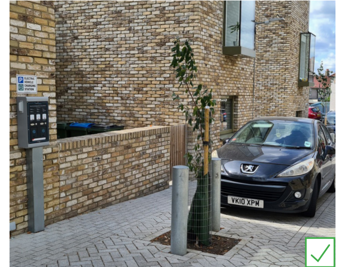
Example of a well-integrated wall-mounted electric vehicle charging meter
