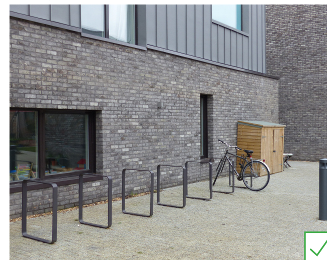
Example of a simple contemporary public cycle parking facility
