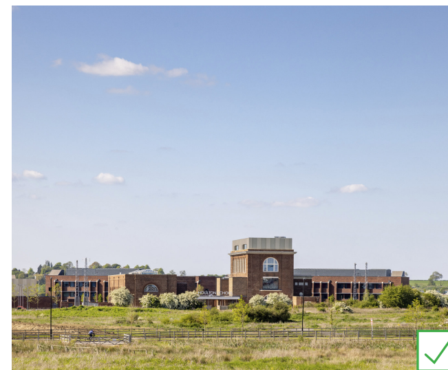
Distinct local Landmark Buildings help with wayfinding and orientation and enriches the place
