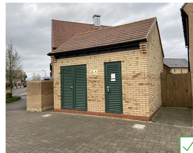
Substation enclosed in a brick structure which is in keeping with the adjacent built form
