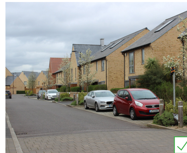
Sensitively integrated visitor parking with well-planted verges
